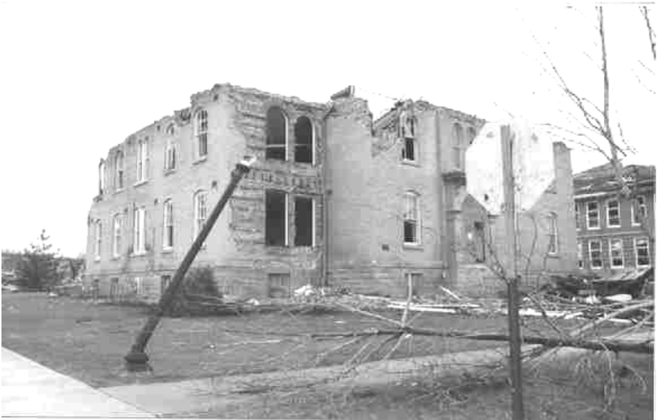
"Old Main" in St. Peter, MN. Damaged by the March 29th tornado. This is an example of the F3 damage done that day..
